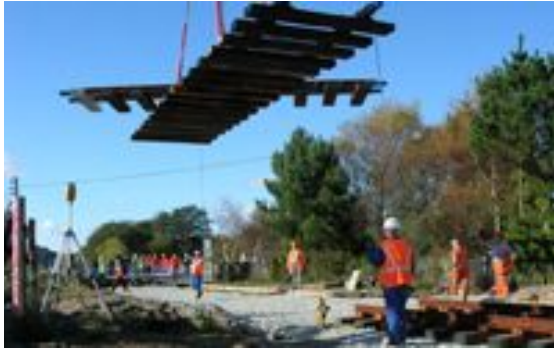
Installing the Cambrian Crossing
