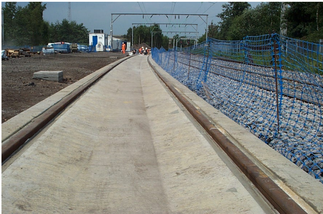
Balfour Beatty slab track installation on Crewe-Kidsgrove line
