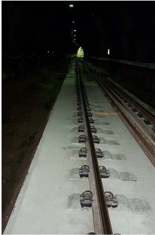
Rheda concrete slab track in Prestbury Tunnel
